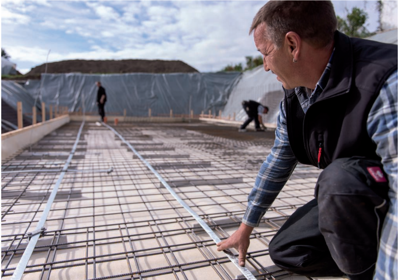
Installing a foundation earther
